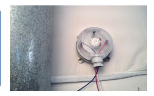
2. Drill 9/32" (7mm) hole in kitchen range hood exhaust duct. Install pressure tap with supplied sheet metal screws.
