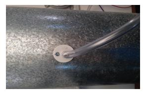
3. Attach supplied vinyl tubing to pressure tap and to lower port on RangeRelief Pressure Switch.
